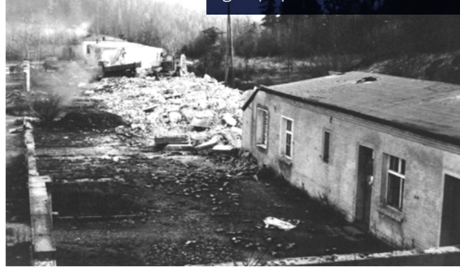
Demolition of the former detention building, 1964
