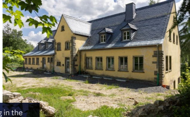
Transfer of the former quarry administration building to the Bavarian Memorials Foundation in 2023 (photo from 2019)
